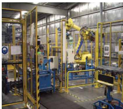
Production at Hirotec is largely automated to ensure a consistently high standard in the parts produced.
